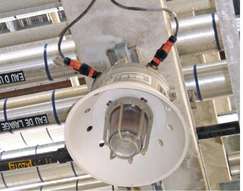
**GESIS®**HAZLOC connectors easily integrate with existing I,C,E devices providing the option to prefabricate light fixtures, RTDs, and other devices for a fully pluggable system. Quickly disconnect for fast change-outs that reduce downtime. Factory integration of connectors to devices is easy and no customization of the device is required!
